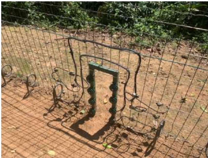
Figure 25: Image of a typical 'critter gate' to be installed in the fence surrounding the development footprint.
