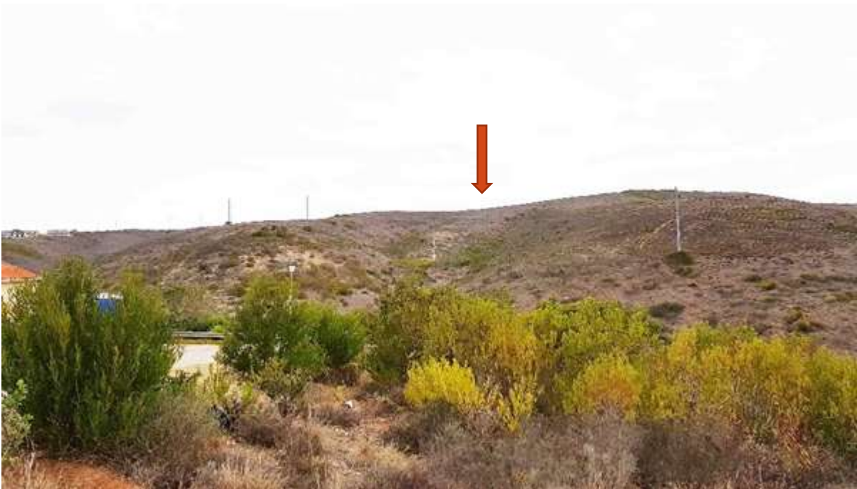
Figure 34: View from within Hartenbos Heuwels towards the North overlooking the ridgeline and powerline (Source: BCK 2022).
