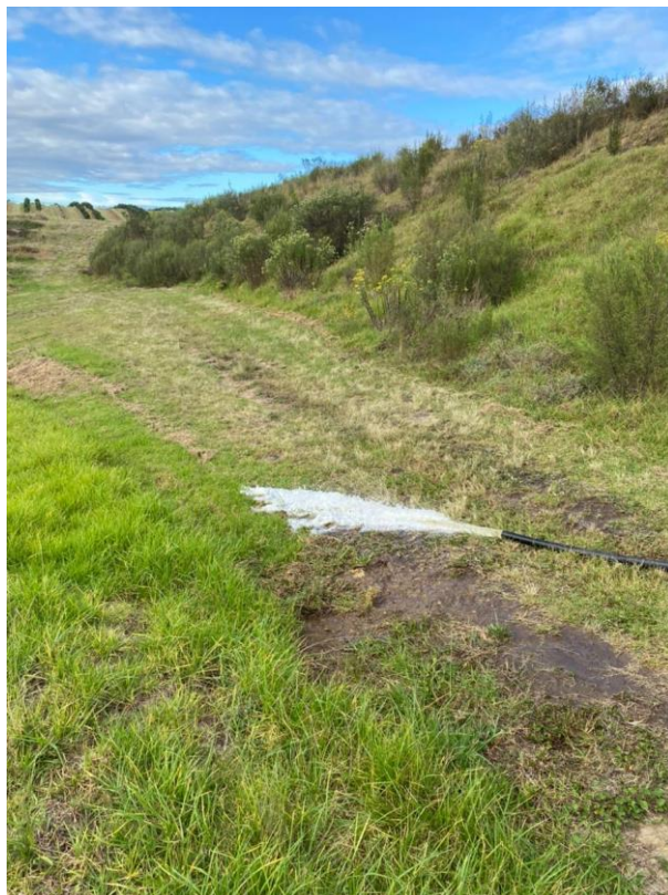
Figure 4. Water discharged over a grassed embankment to avoid erosion of the stream bed and banks.
