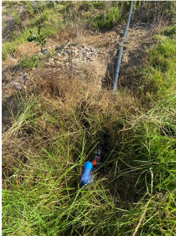
Figure 3: HDPE pipe installed to pump water out of the dam.
