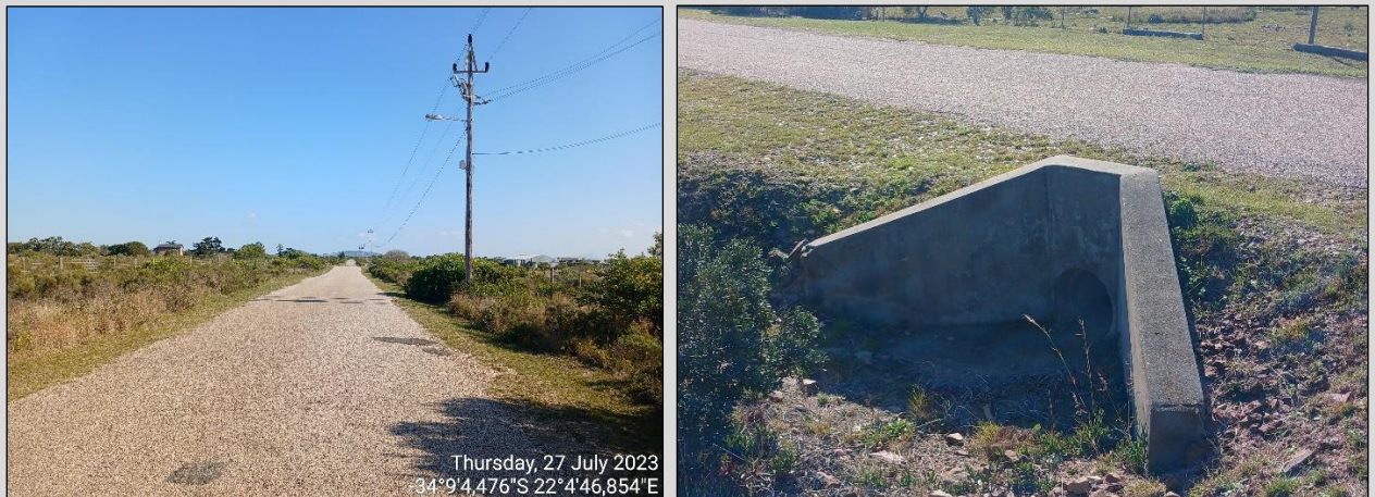
Figure 7: Left photograph – Klipheuwel Road. Right photograph – existing Municipal culvert.
