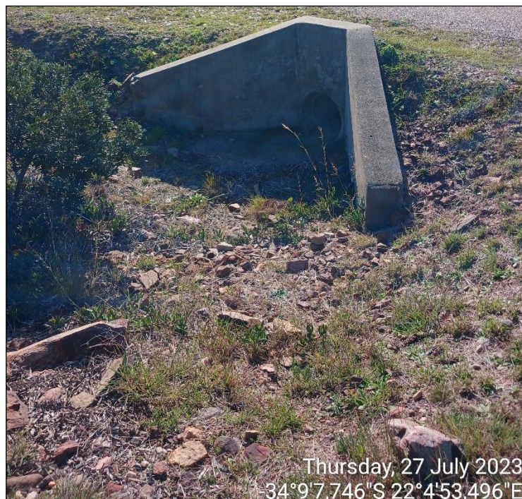
Figure 4: Existing Municipal Culvert adjacent to Ptn 209 of Farm 220, Aalwyndal.
