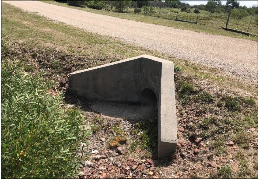
Figure 13: Culvert on the eastern boundary of the site underneath Klipheuwel Road
