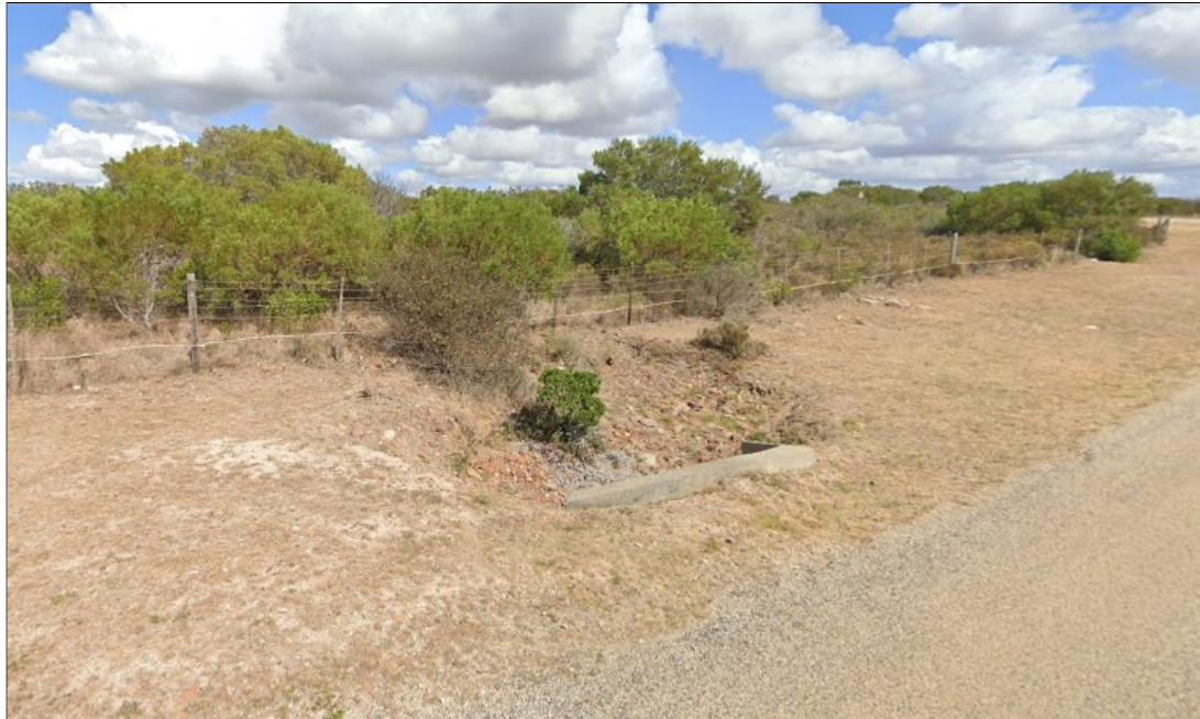
Figure 12: Culvert on eastern boundary underneath Klipheuwel Road.
