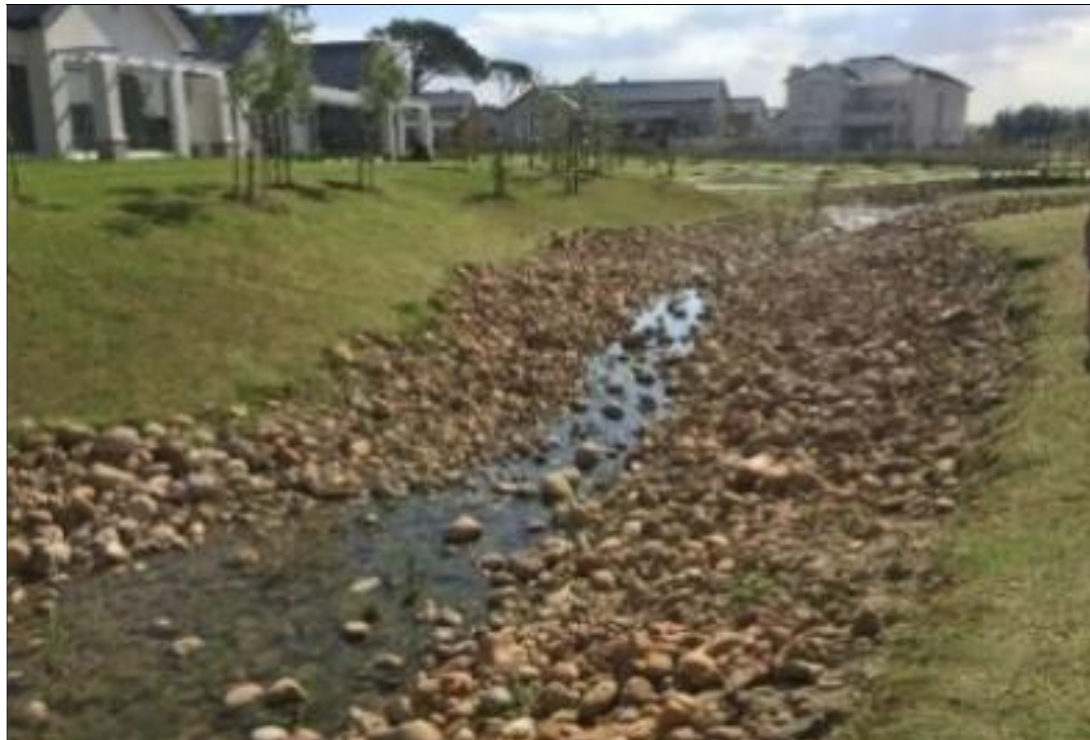
Figure 5: Example of swales
