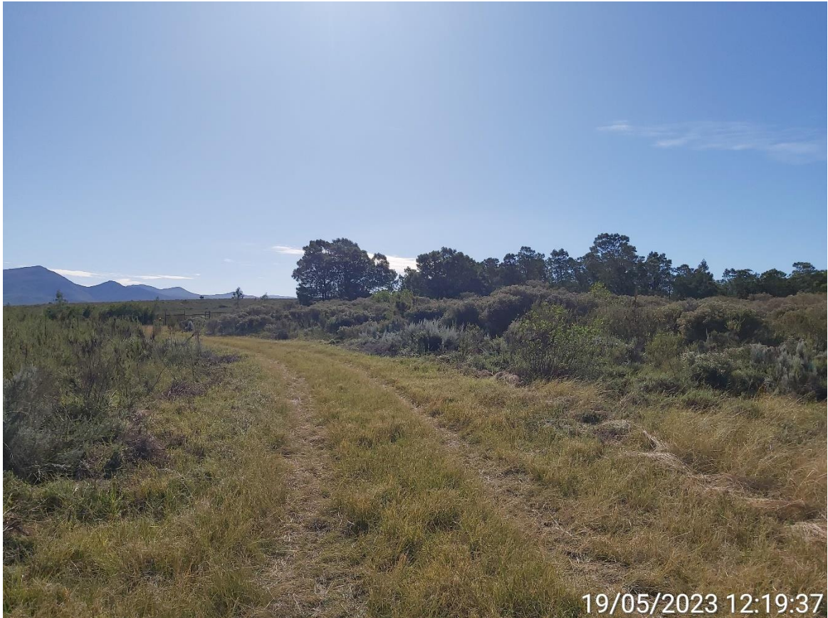
Figure 3: Access Road on Portion 1 of Farm 172, near Herbertsdale.
