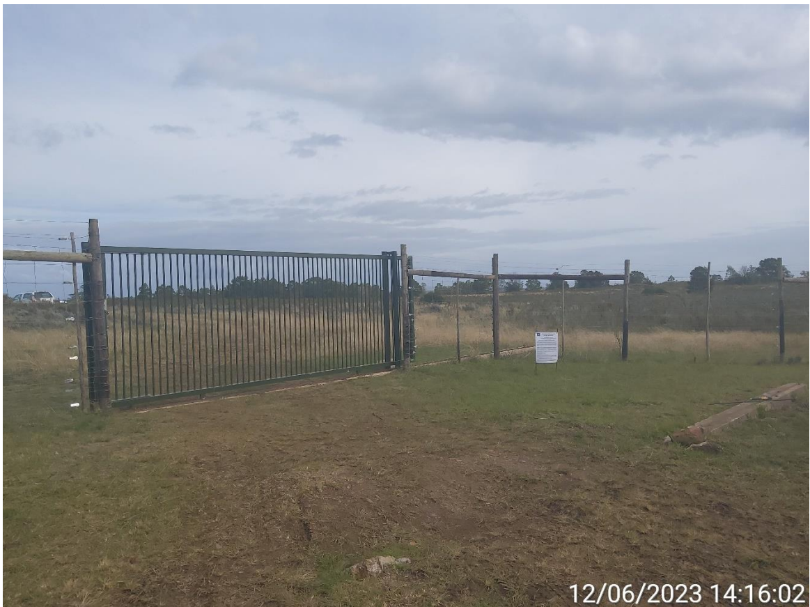
Figure 2: Main Entrance at Portion 1 of Farm 172, near Herbertsdale.
