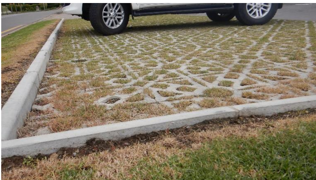
Figure 17: A local example of the use of open pavers for car parking in George.
