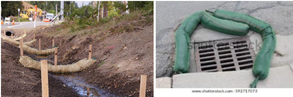
Figure 16: Examples of silt socks placed perpendicular to the flow of water. These reduce the force of water flow, erosion, and can prevent unwanted sedimentation on the site.
