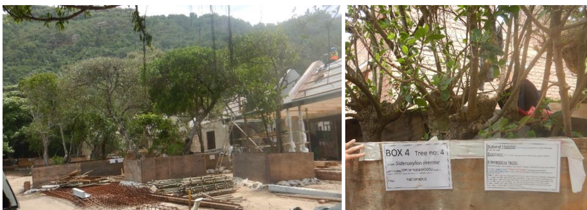
Figure 14: An example of a construction site with protected and other indigenous trees marked and sectioned off from the rest of the construction site. Each tree and box was marked, and interesting facts about the species and its ecology was provided on the construction site.
