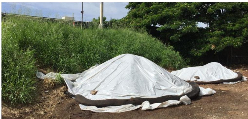
Figure 19: An example of a protected stockpile (image from stormwaterhawaii.com).
