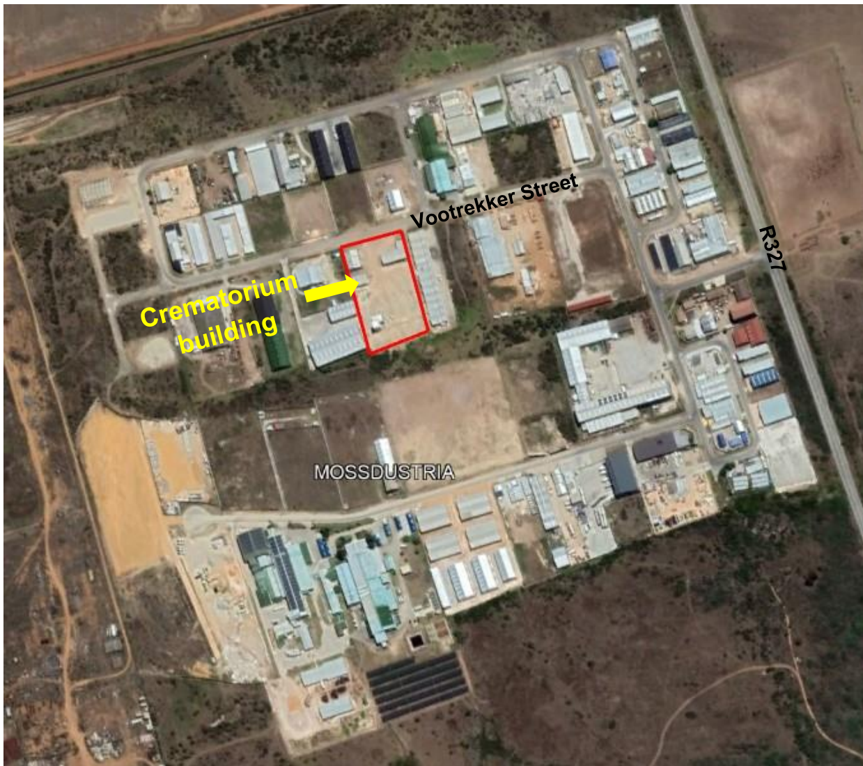
Figure 1: Erf 50 (red outlined area) situated in MossDustria (Source: Google Earth, imagery date 20/11/2022)
