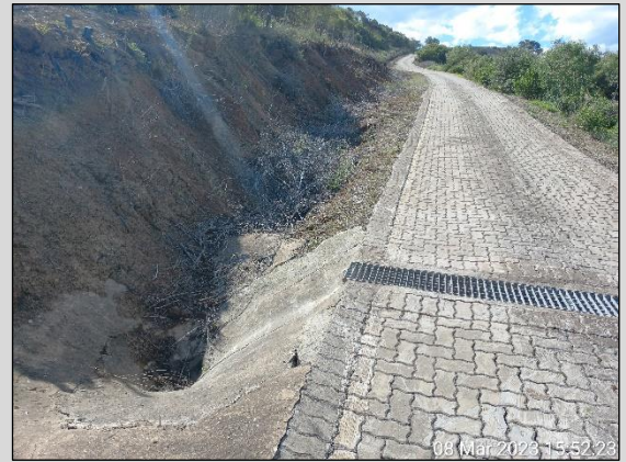
Figure 28: Existing stormwater channel, consisting of grass blocks, on RE/2833. Existing soakaway in access road.
