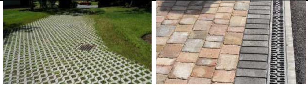
Figure 1: Example of permeable driveways (left) & soakaways (right).
