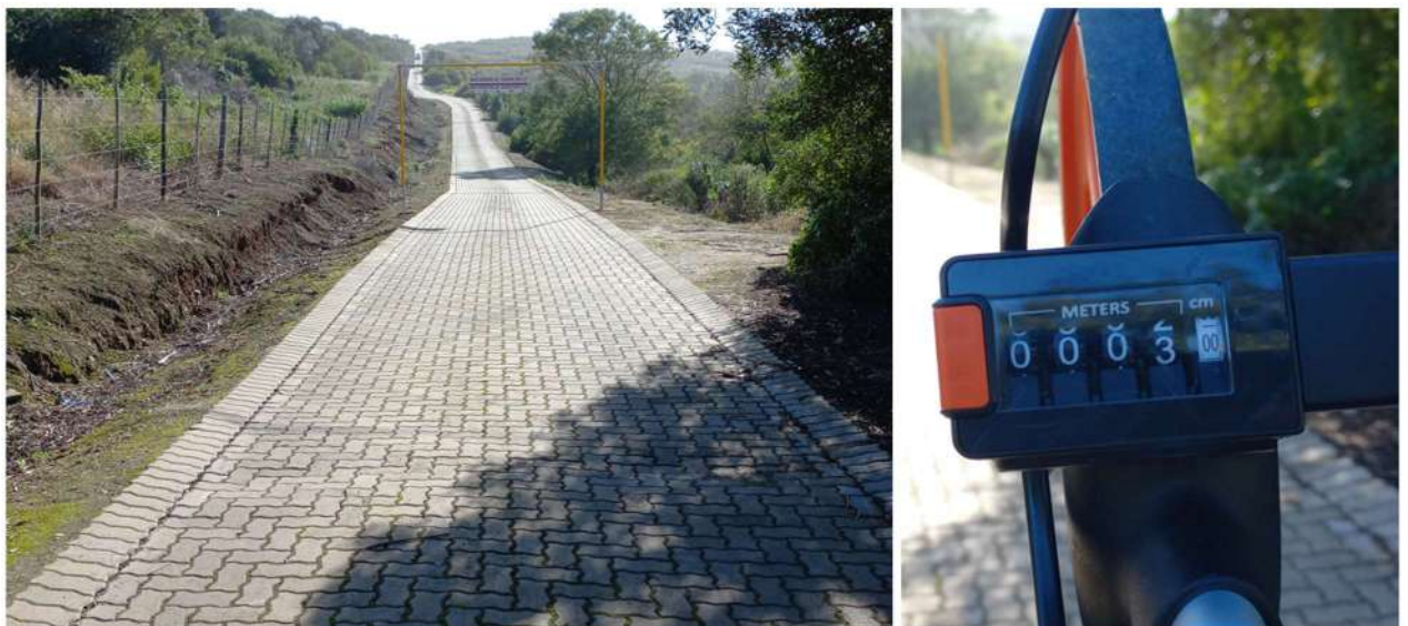
Figure 8-5 - Existing Servitude Road
