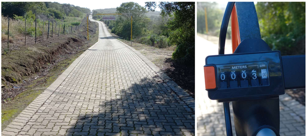
Figure 8-5 - Existing Servitude Road
