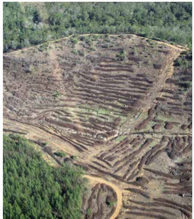
Cleared material stacked along contour lines. © Saskia Fourie / WWF
