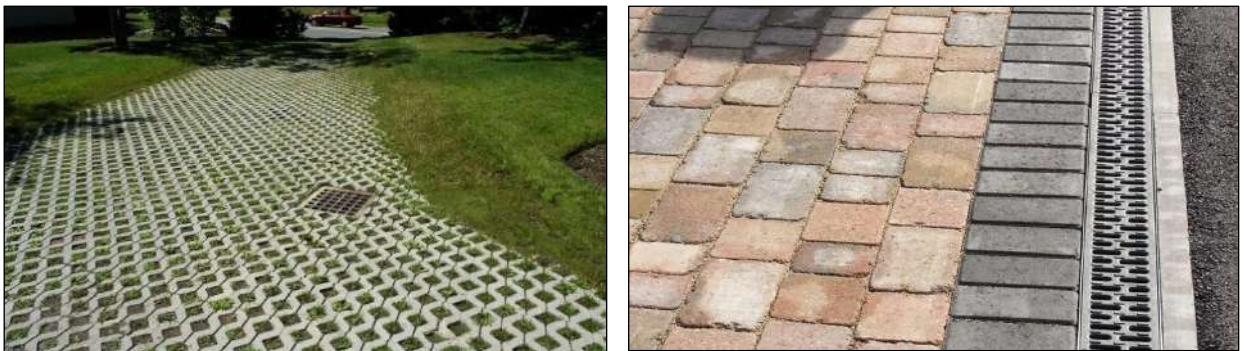
Figure 4: Example of permeable driveways & soakaways.
