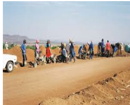
Figure 7 Gravel road built with Hyson Cells.
