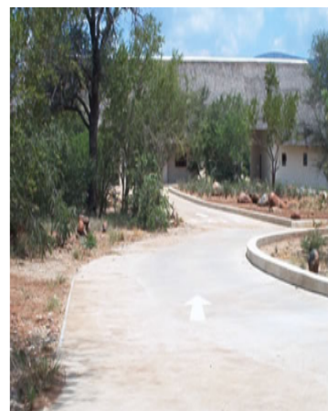
Figure 7 Gravel road built with Hyson Cells.
