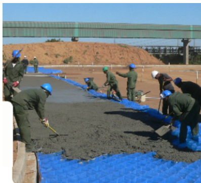
Figure 6 Hyson Cells filled with concrete
