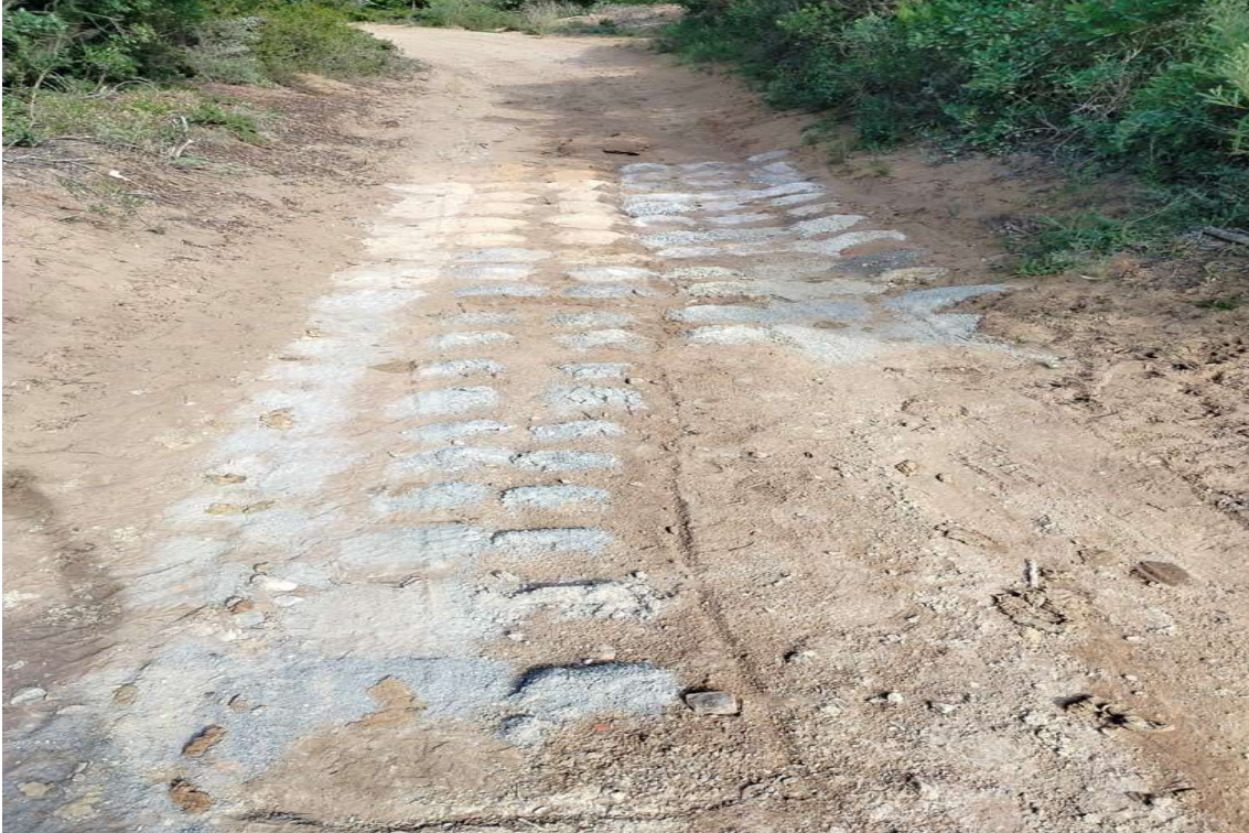
Photo 1: One-meter interval drill chips displayed by drilling contractor
