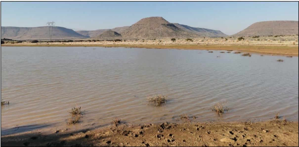
Figure 4-6: An artificial system including an impoundment in the project area (August 2023)
