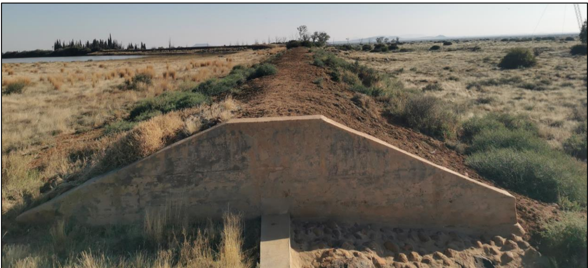
Figure 4-8: An impoundment located in the upper reaches of HGM1 (August 2023)
