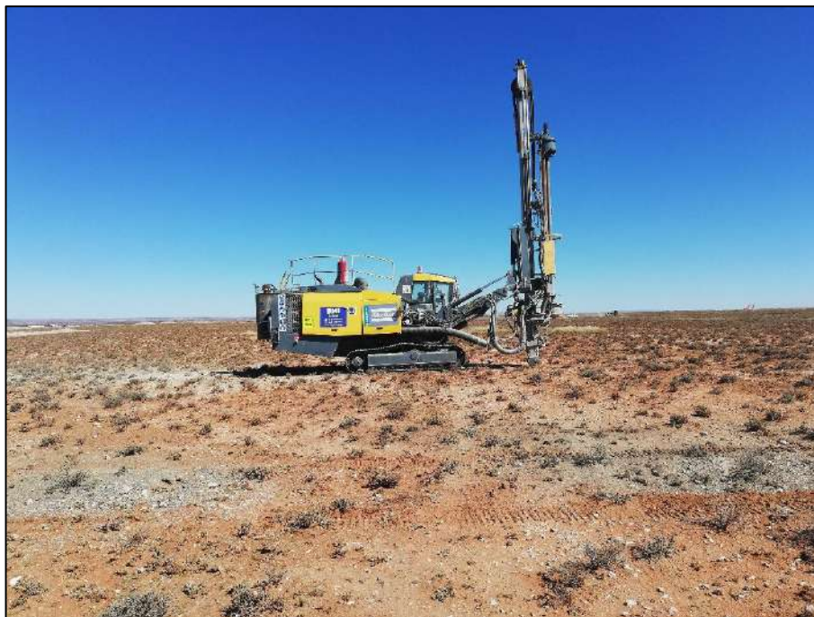
Figure 8: Pre-drilling of holes prior to the ramming of steel piles.
