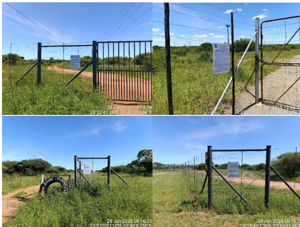
Figure 92: Site Notice board placed at various positions along the boundaries of the affected properties.
