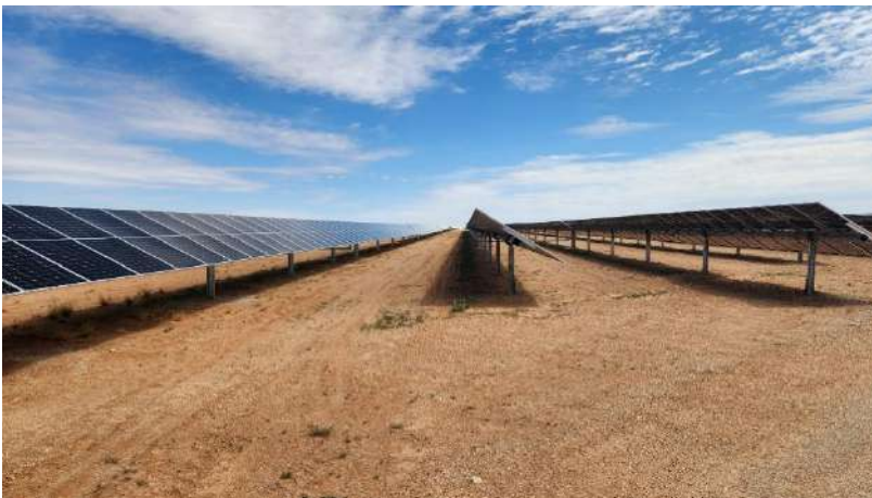
Figure 7: Example of Single Axis Tracking Technology (Cape EAPrac, 2024).
