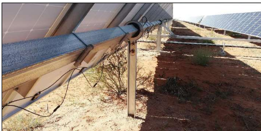
Figure 11: Completed ramming and assembly showing vegetation remaining intact beneath the modules.
