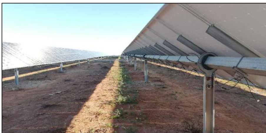
Figure 12: Showing vegetation re-establishing along the driplines of the arrays within weeks after installation.
