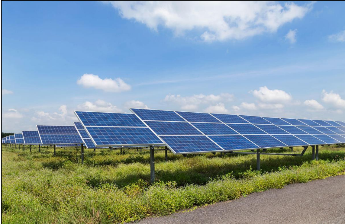
Photograph 1.1: Typical PV SEF facility
