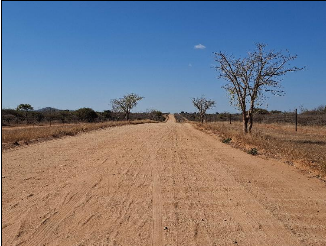
Photograph 3.4: View along Mogwadi/Bottelier Road looking west
