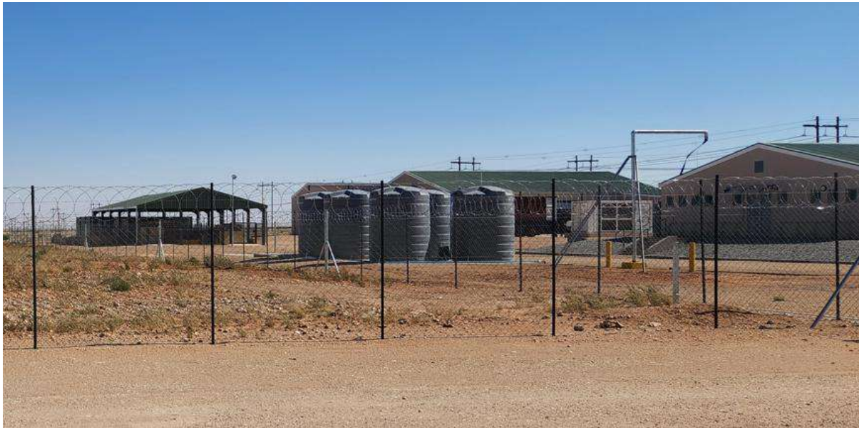
Figure 12: Example of typical newly constructed Auxiliary building with offices, warehouse, store and rainwater storage (Photo: Cape EAPrac, 2024).
