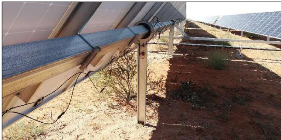
Figure 10: Completed ramming and assembly showing vegetation remaining intact beneath the modules.
