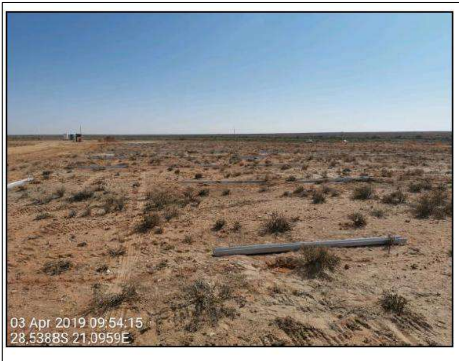
Figure 8: pre-drilled holes are backfilled with a wet sand mixture and steel piles placed in position ready for ramming.
