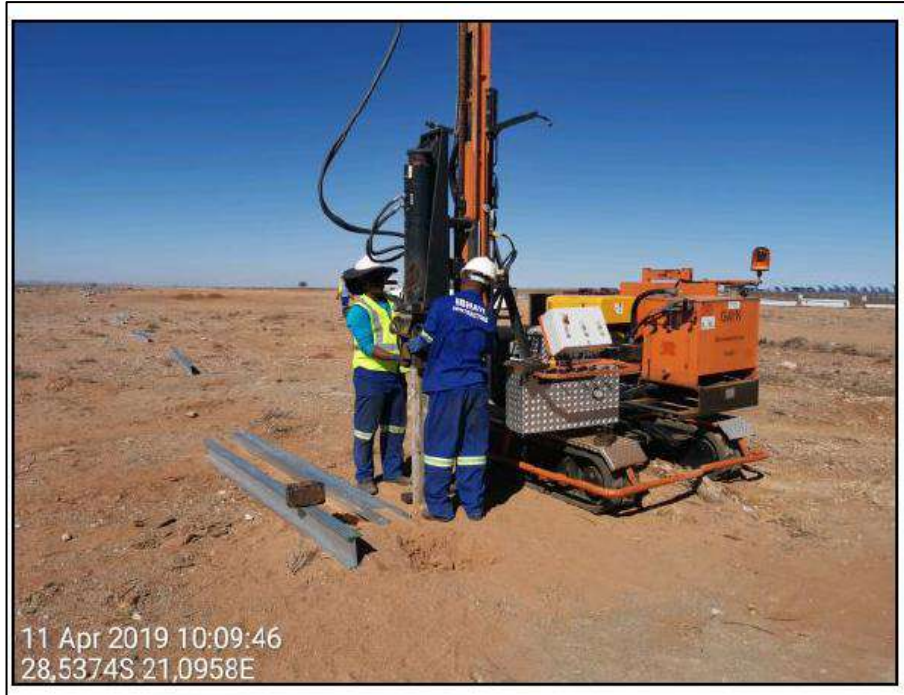
Figure 9: Ramming of steel piles into the pre-drilled / backfilled holes.
