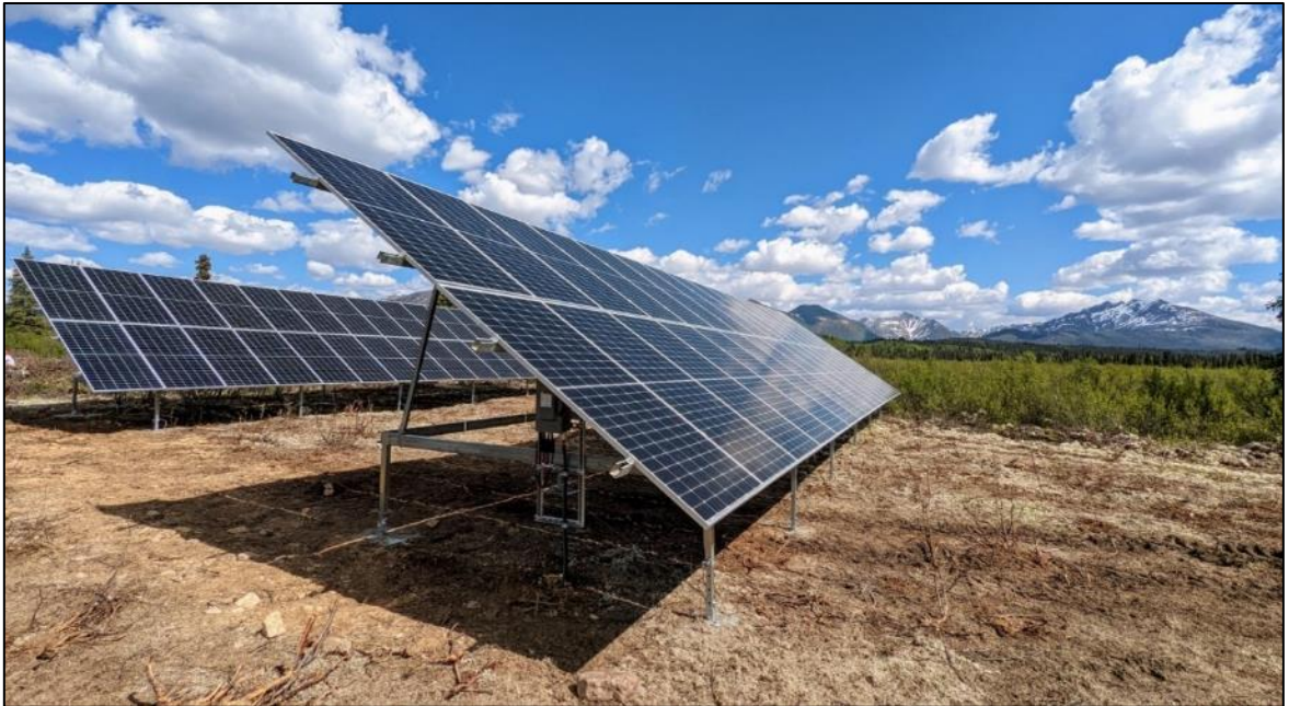
Figure 3: Photographic example of what the proposed PV could look like as fixed and single portrait model on a tracker.
