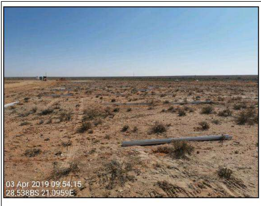
Figure 9: Pre-drilled holes are backfilled with a wet sand mixture and steel piles placed in position ready for ramming.
