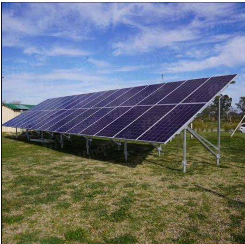
Figure 6: Example of Earth Screw Mounting Technology (HQ Mount, 2023).
