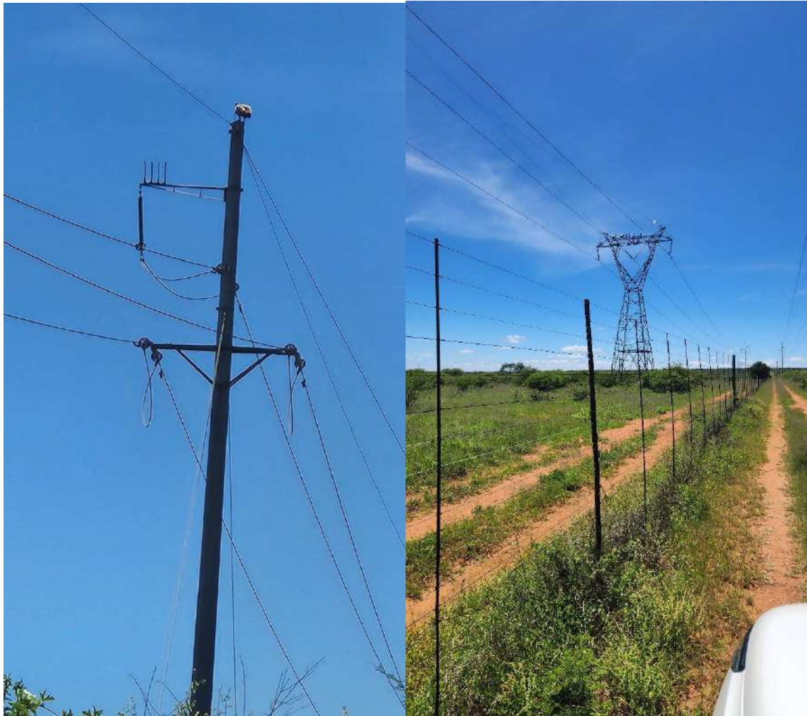
Figure 23: Photographic examples of existing Eskom Grid Infrastructure on and adjacent to the study site.
