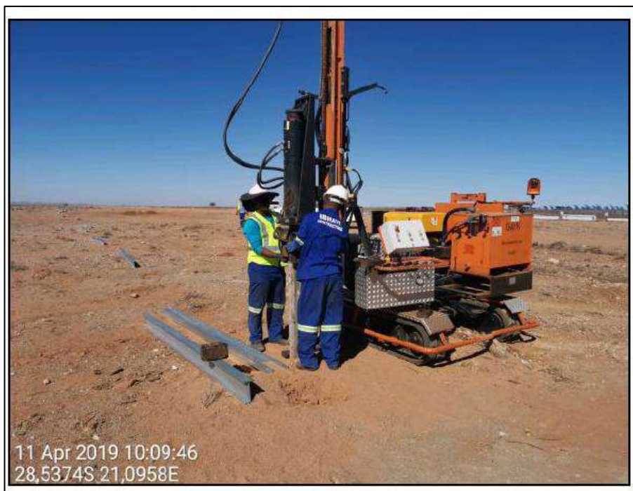
Figure 10: Ramming of steel piles into the pre-drilled / backfilled holes.
