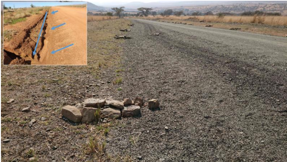
Figure 4-2 Example of road margin erosion prevention.
