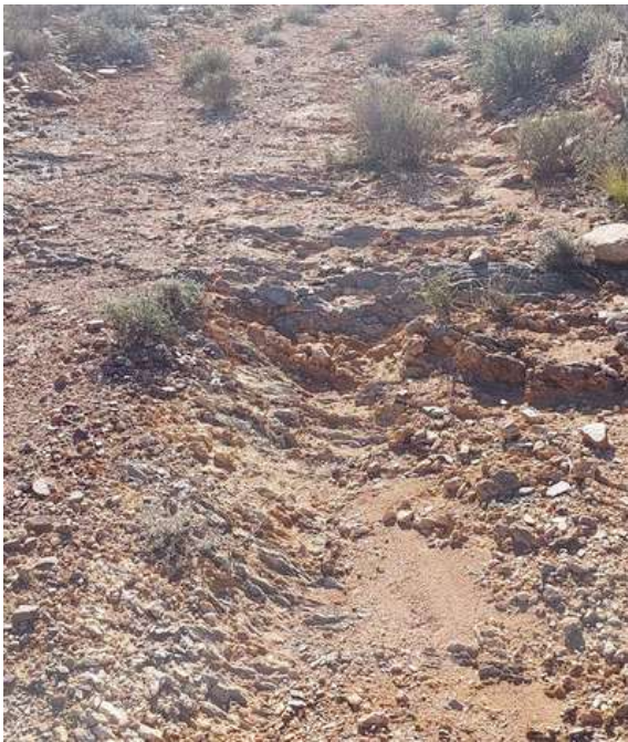
Photo 7: Taken at Ch 3300.
