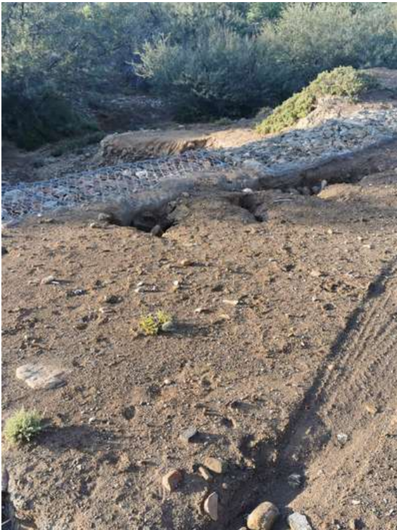
Photo 3: Taken at ch. 150
