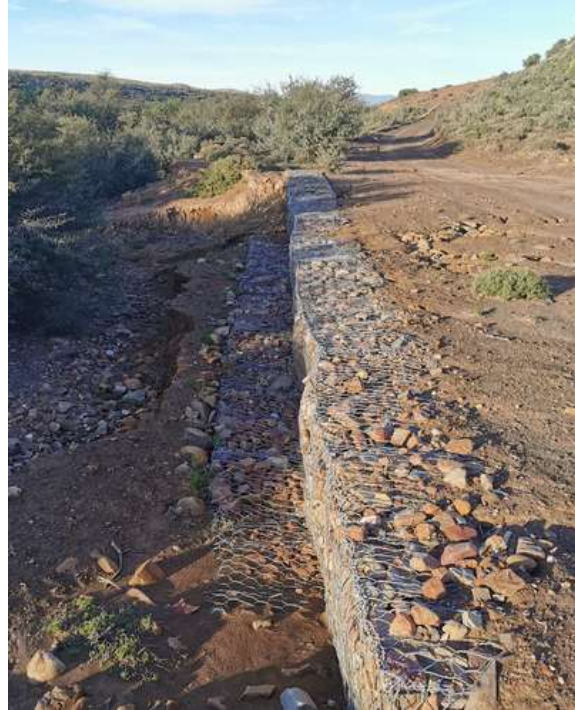
Photo 3: Taken at ch. 150
