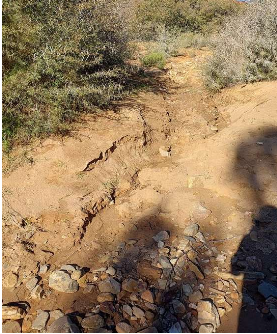
Photo 5: Taken at Ch 2340 (stream crossing)
