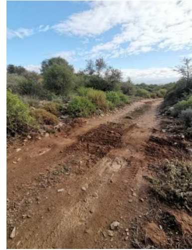
Figure 11: photo 35, The road exhibits natural firmness and is in moderate condition.
