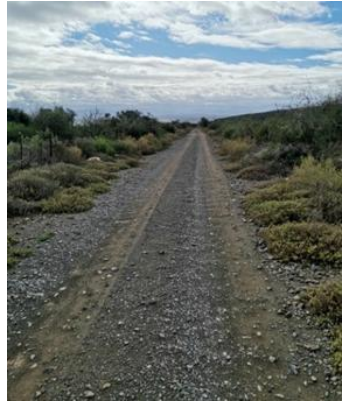
Figure 16: photo, 56 The road exhibits natural firmness and is in moderate condition.
