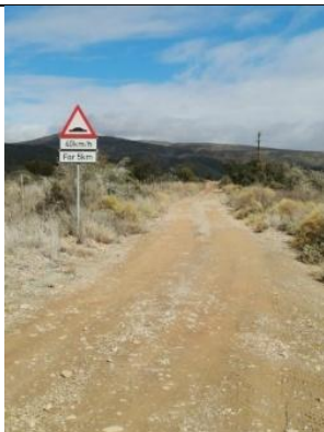
Figure 21: photo 72, the road exhibits natural firmness and is in moderate condition.
