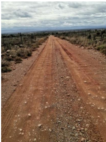
Figure 18: photo 67, The road exhibits natural firmness and is in moderate condition.
