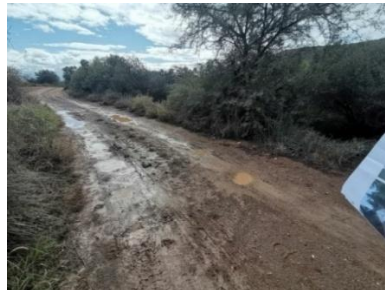
Figure 13: photo 43, filled watercourse culverts needed.
