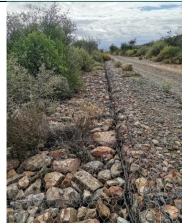
Figure 14: photo 51, watercourse area with gabion mattresses.
