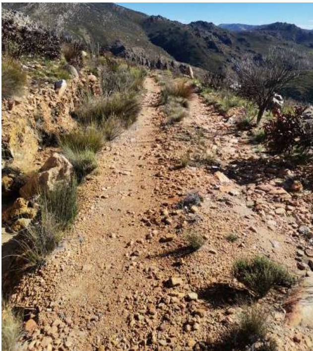
Figure 25: Photo 84, road in good condition. Reshaping of humps required.
