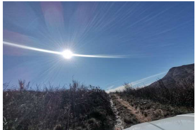
Figure 6: Photo 6, road eroded. Imported fill material along wheel tracks required.
