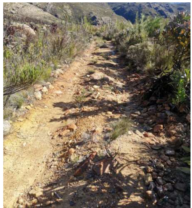
Figure 26: Photo 87, road in average condition. Reshaping of humps required.
