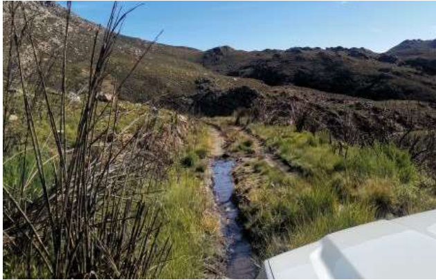
Figure 27: Photo 90, road is in average condition. There's standing water on wheel tracks due to poor stormwater drainage.
