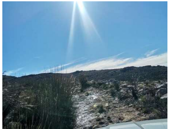
Figure 10: Photo 18, road in average condition. Weathered wheel tracks with a lot of exposed rocks.
