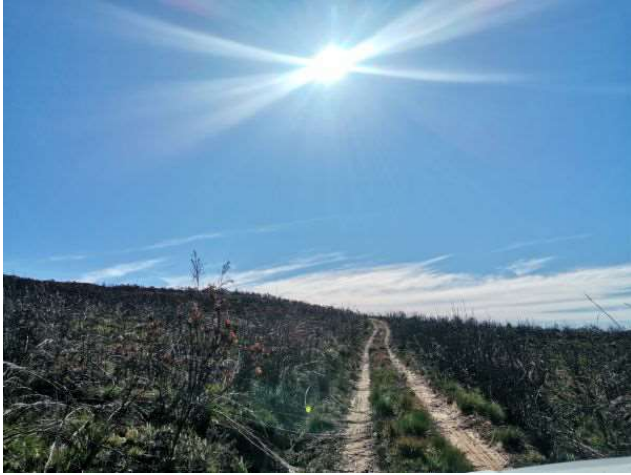
Figure 7: Photo 7, road path is in excellent condition, no remedial work required.
