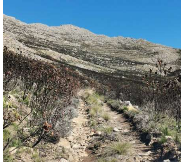
Figure 4: Photo 3, the road is in average condition with erosion along wheel tracks. Imported material required.
