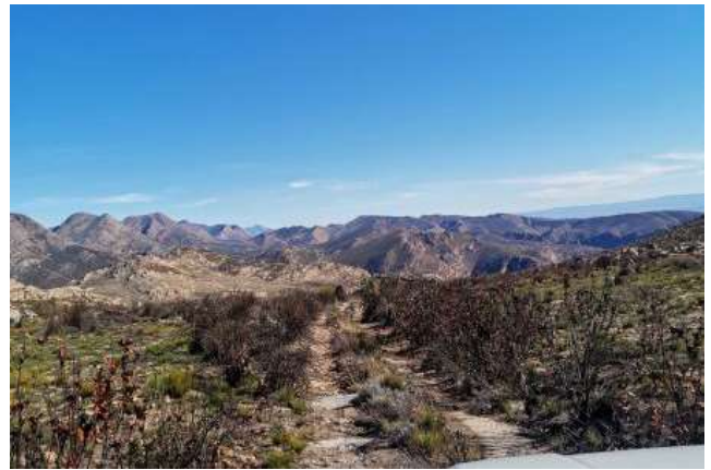
Figure 12: Photo 24, the road is in average condition, slightly eroded
