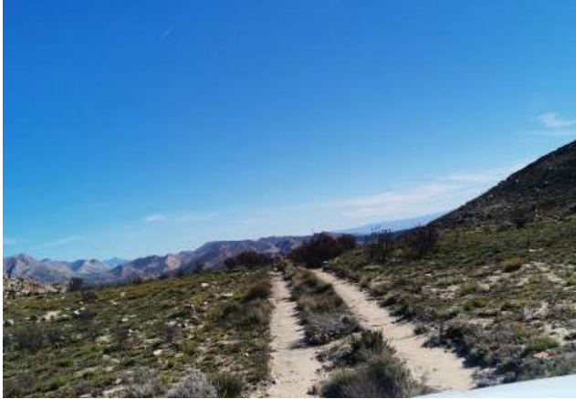
Figure 11: Photo 23, road in good condition. Bumps need reshaping.
