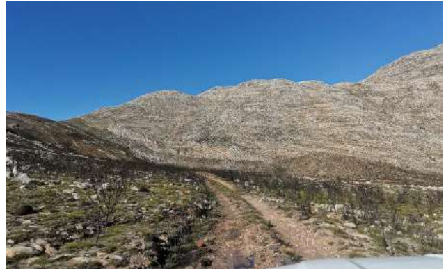
Figure 16: Photo 48, the road is in good condition. No remedial work required
