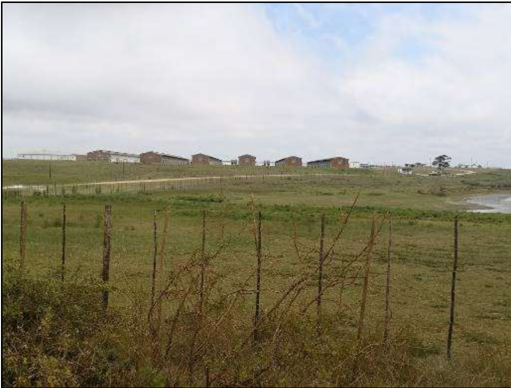
Photograph 2: Existing laying houses
