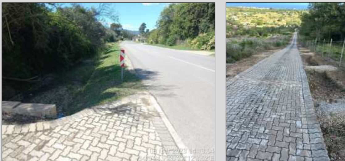
Figure 6: Access directly off Sandhoogte Road.
