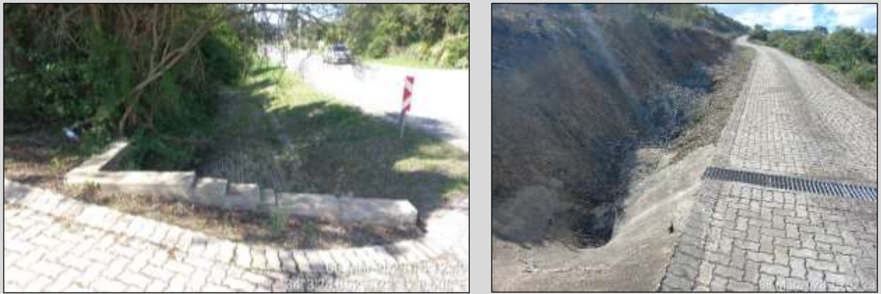
Figure 27: Existing stormwater channel, consisting of grass blocks, on RE/2833. Existing soakaway in access road.
