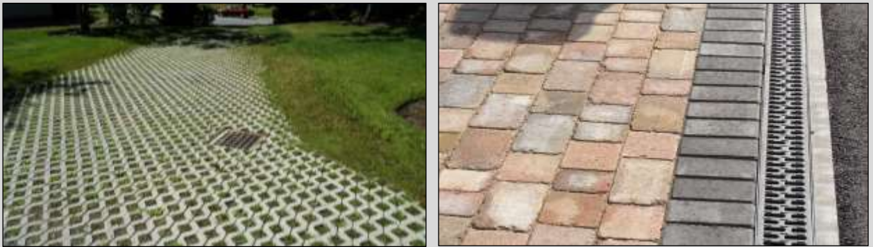
Figure 26: Example of permeable driveways & soakaways.
