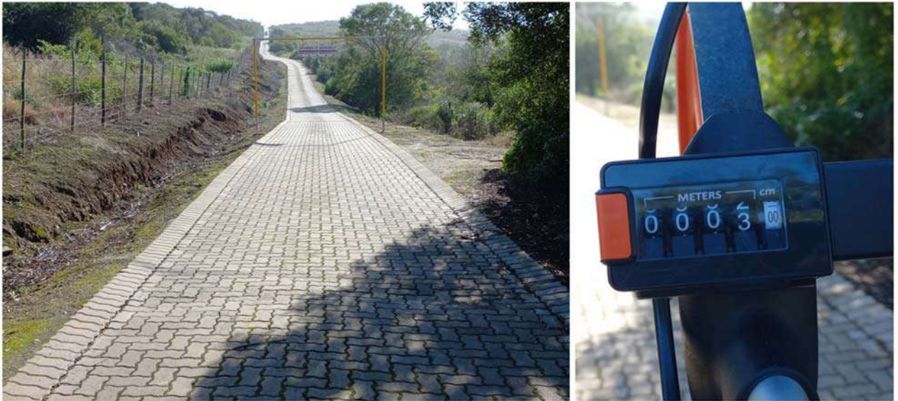
Figure 8-5 - Existing Servitude Road
