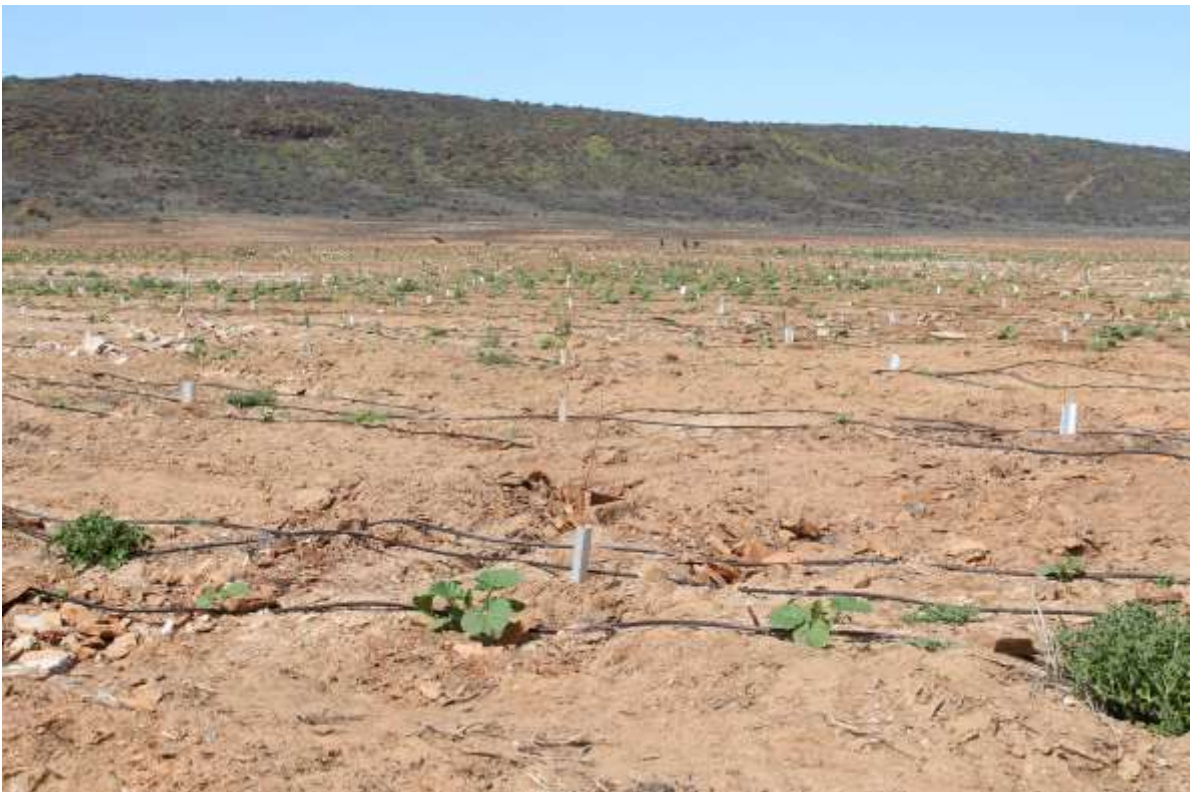
Figure 10: Initial site photographs post clearing and planting of trees.
