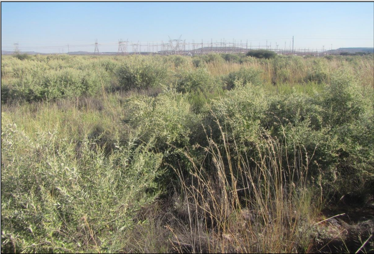
Looking southwest towards the Ferrum Substation (Orton, 2024).
