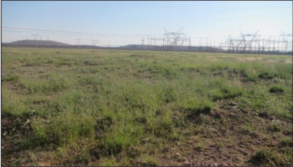
Looking west towards the Ferrum Substation (Orton, 2024).
