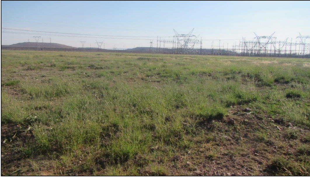
Figure 9: Looking west towards the Ferrum Substation.
