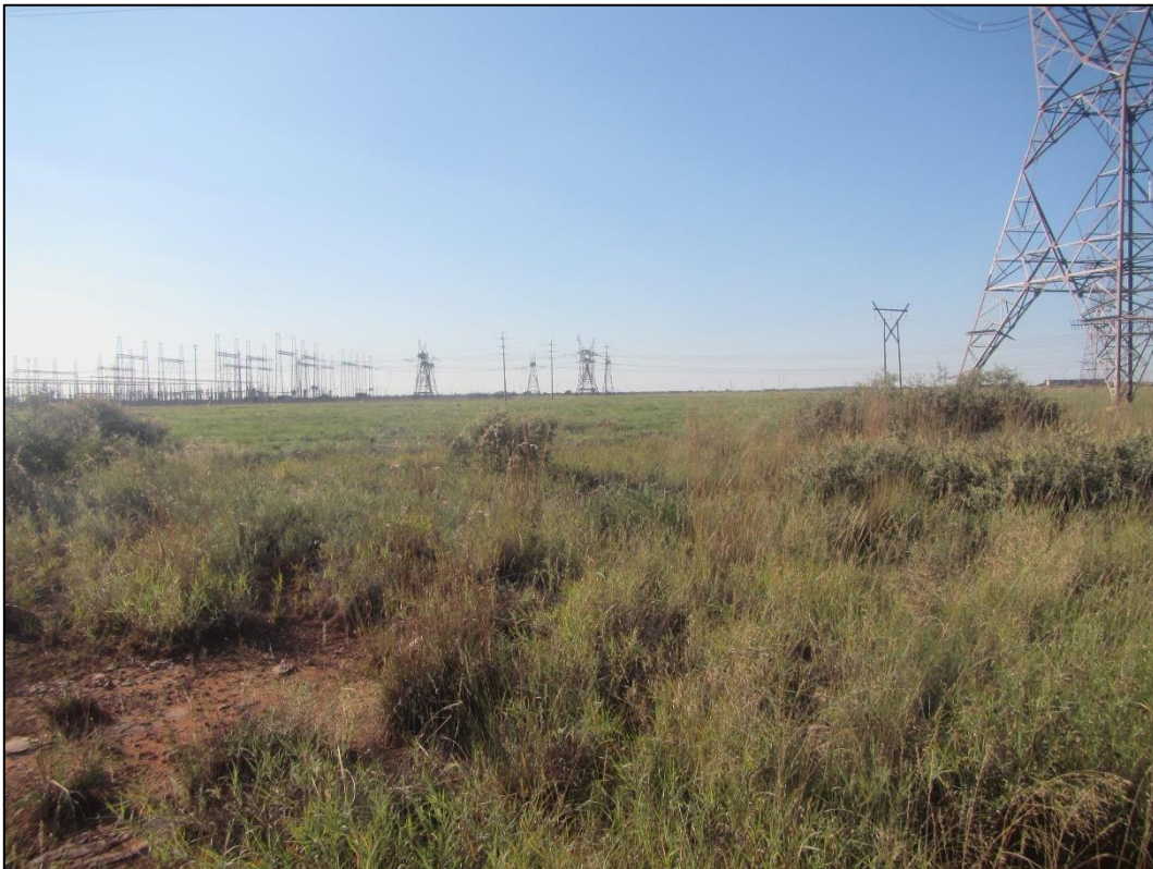
Figure 13: Looking north towards the Ferrum Substation.
