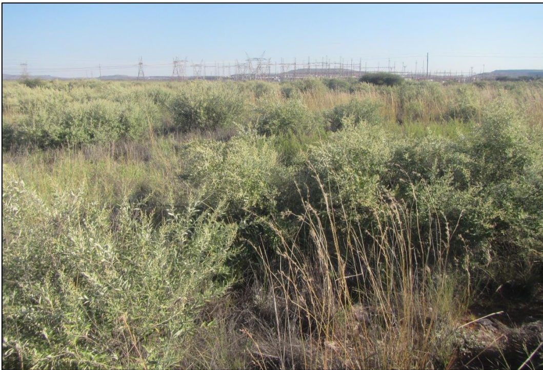
Figure 11: Looking southwest towards the Ferrum Substation.
