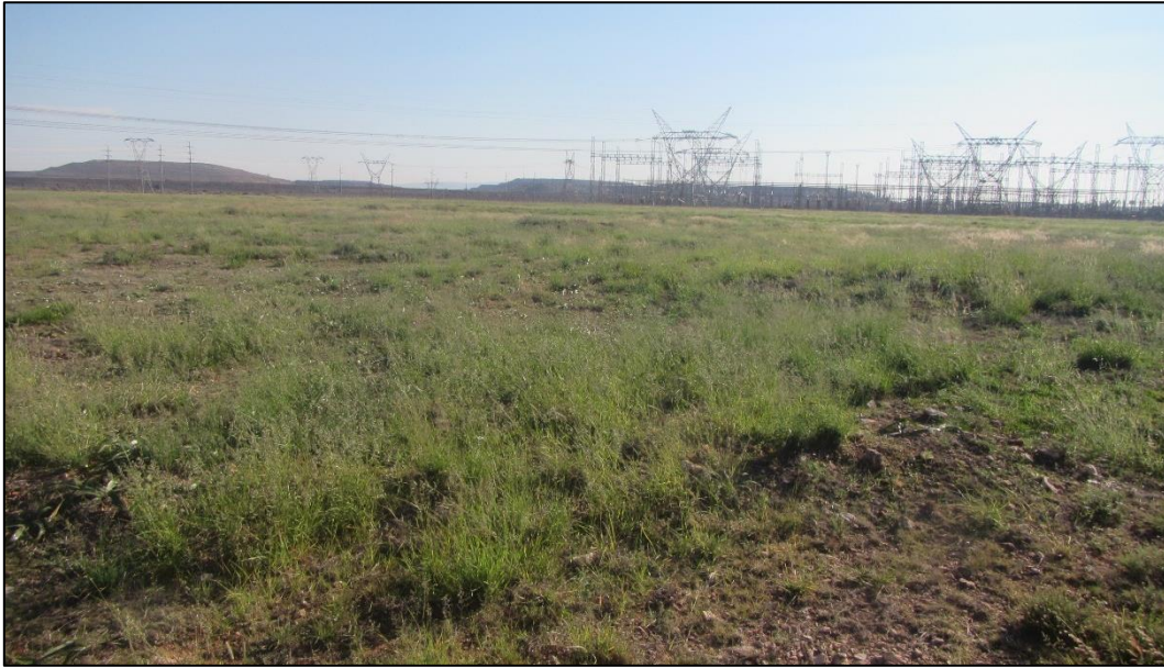
Figure 12: Looking west towards the Ferrum Substation.
