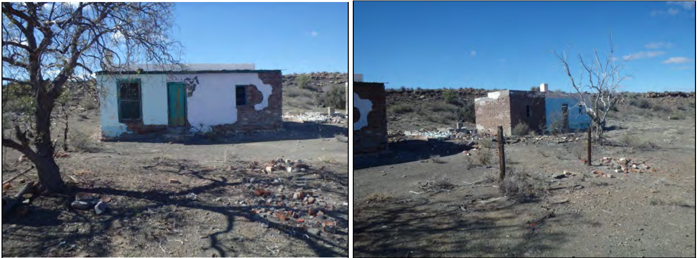
Figure 4.1: Observation BLK055 (Grade IIIC) located approximately 1km from the grid connection corridor
