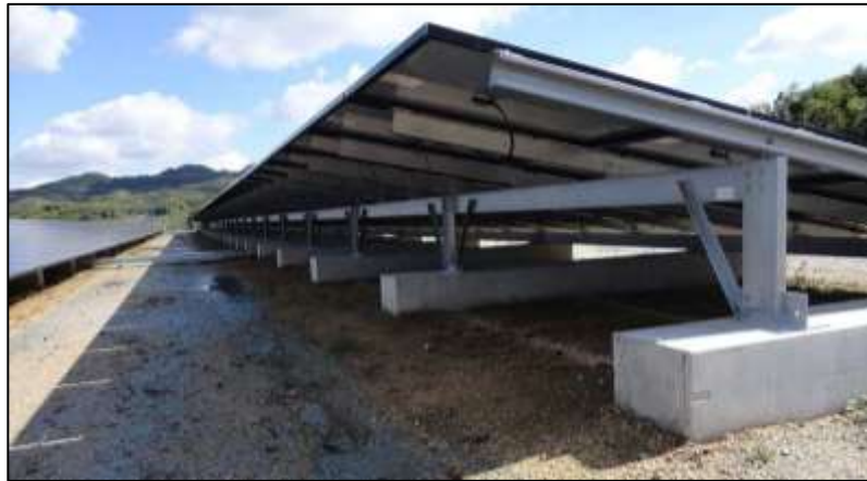
Figure 4: Cast Concrete Foundation
