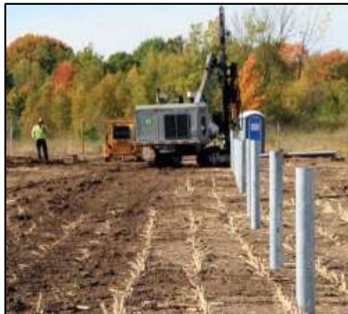
Figure 5: Driven/ Rammed Steel Pile
