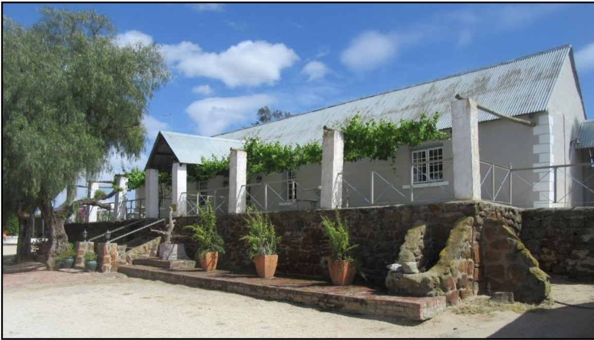
Photograph 3.7: Doornfontein guest facility
