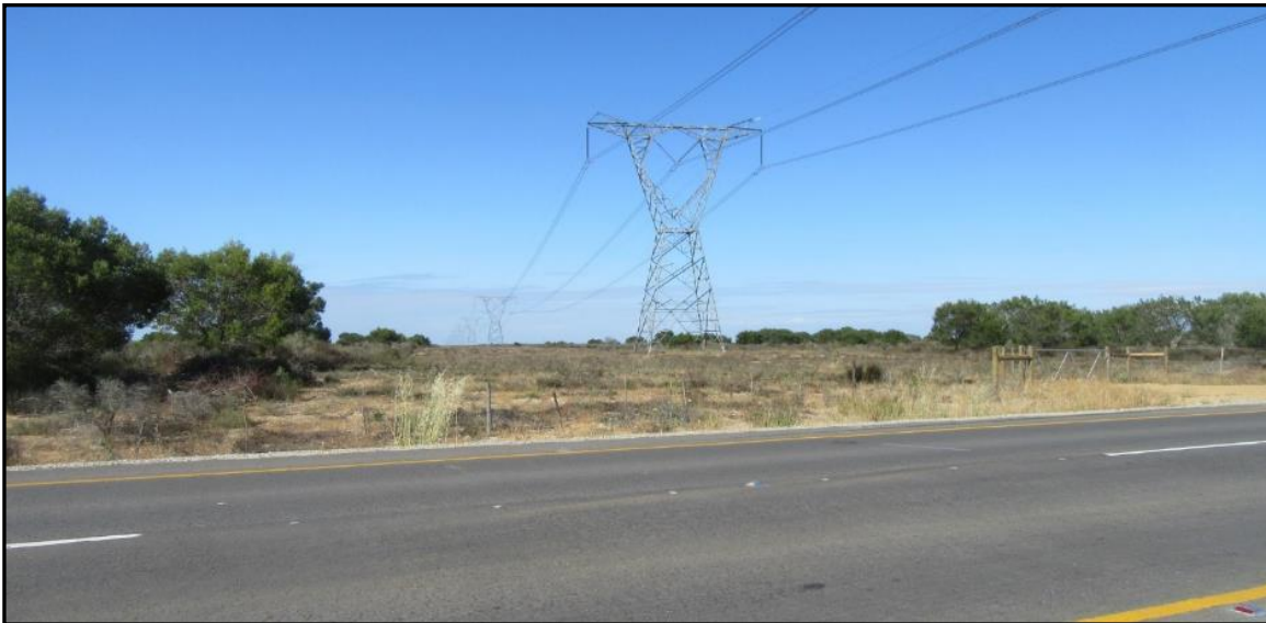
Photograph 3.5: 400 kV line crossing the R399
