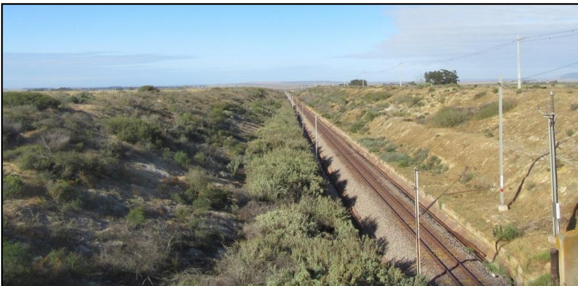
Photograph 3.4: Sishen-Saldanha ore line
