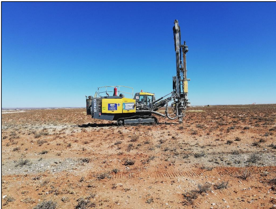
Figure 6: Pre-drilling of holes prior to the ramming of steel piles.
