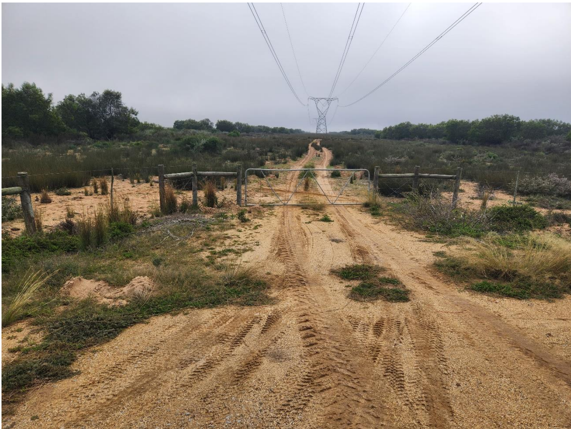
Figure 6: Aurora - Juno 400Kv Powerline crossing the Property
