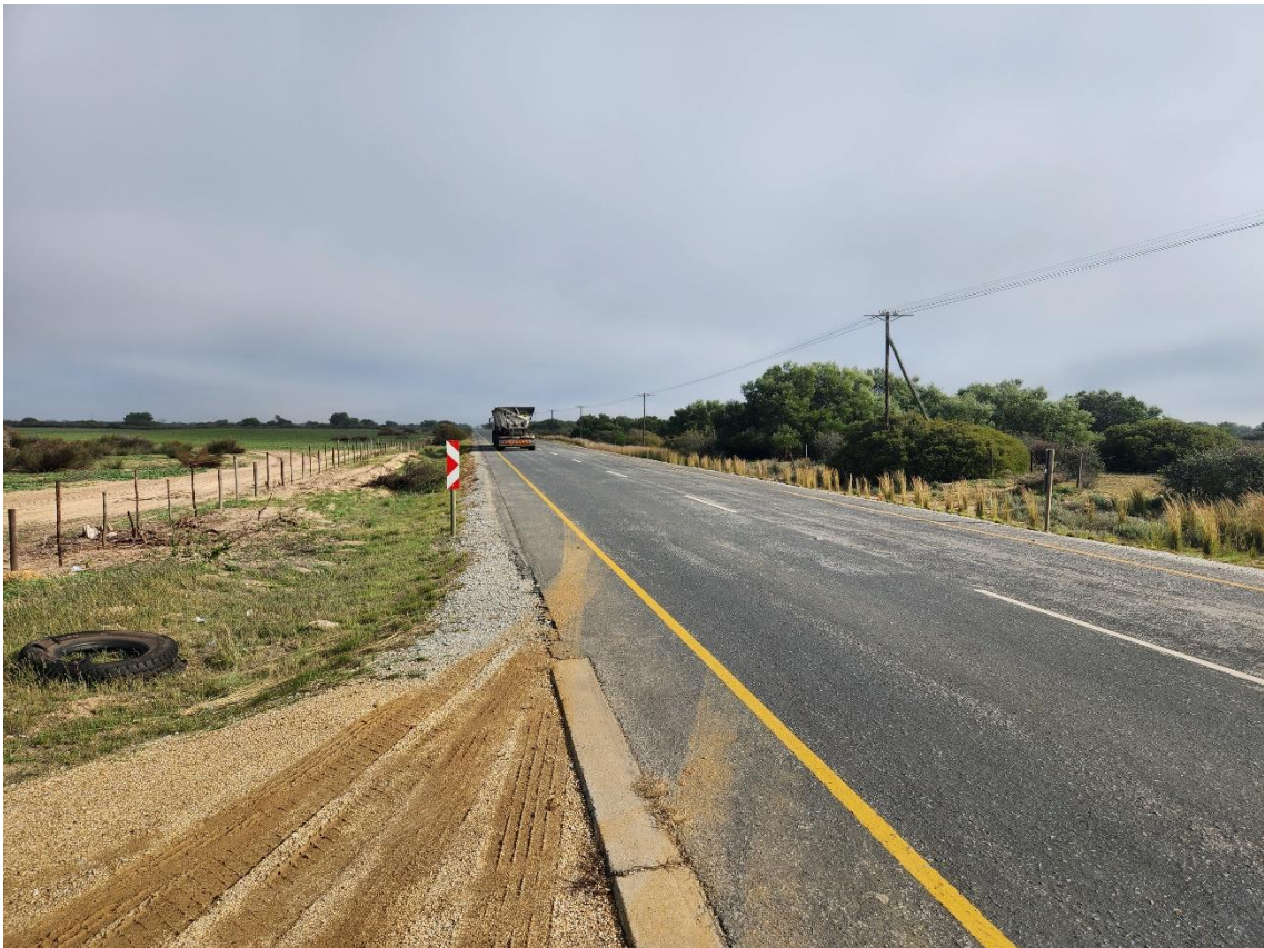
Figure 2: Existing R399 bisecting the Study Site – Orientation East
