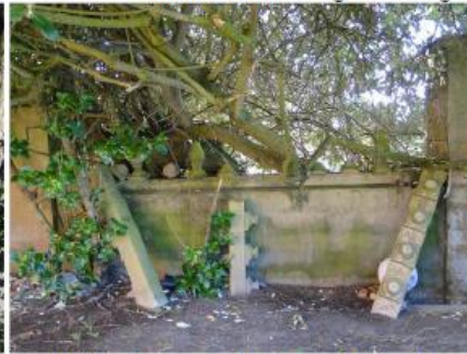
Photos 6-9 (left-to-right): Showing generally dilapidated state of less elaborate historic stonewall presently defining the eastern site boundary.
