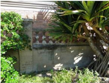
Photos 6-9 (left-to-right): Showing generally dilapidated state of less elaborate historic stonewall presently defining the eastern site boundary.
