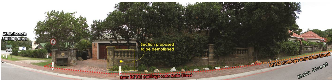
Image 2: South-facing view illustrating section of stonewalling proposed to be demolished as viewed within context of site curilage onto Main Street.
