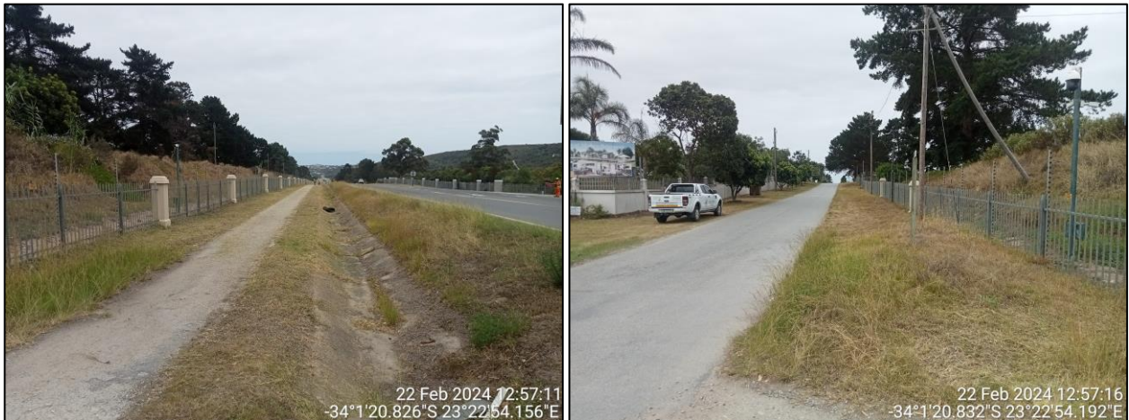
Figure 3: N2 road reserve (left) and Rietvlei Road road reserve (right). Required sewage infrastructure to be installed within the transformed areas of the road reserve.
