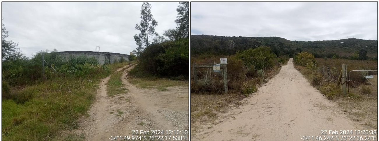
Figure 7: Preferred pipeline route from Goose Valley Reservoir to existing distribution main in N2 road reserve.
