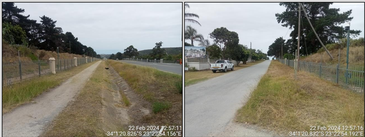
Figure 5: N2 road reserve (left) and Rietvlei Road road reserve (right). Required sewage infrastructure to be installed within the transformed areas of the road reserve.
