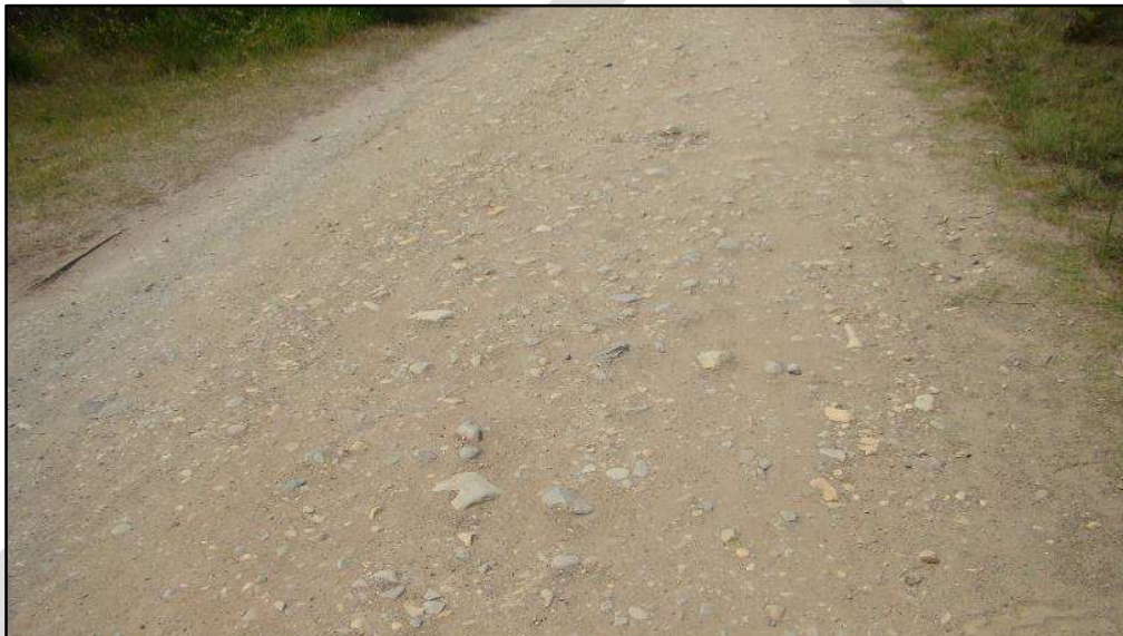
Figure 9: The Rietvlei Road, which runs along the northern boundary of the property, is underlain by beach cobbles
