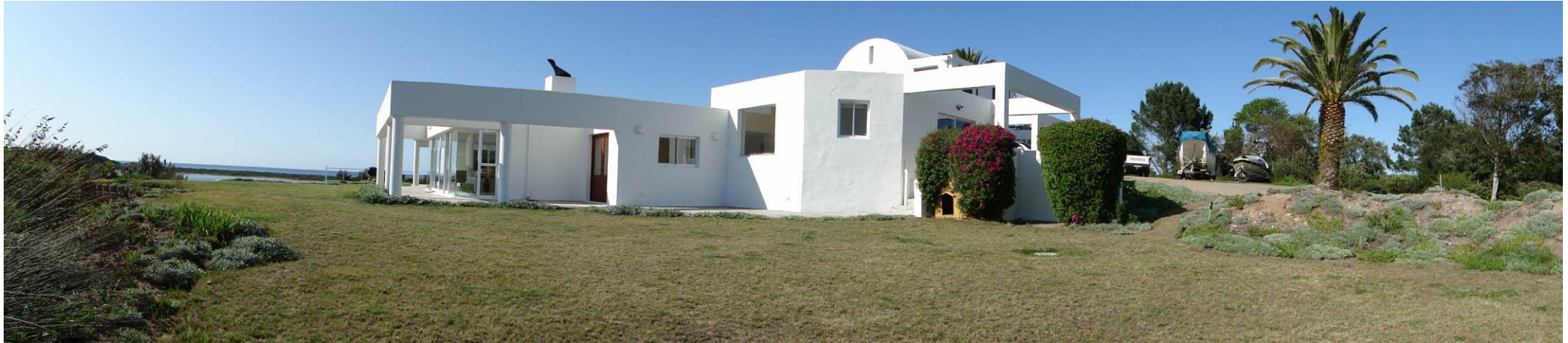
Photo 7: Existing modern main dwelling.
