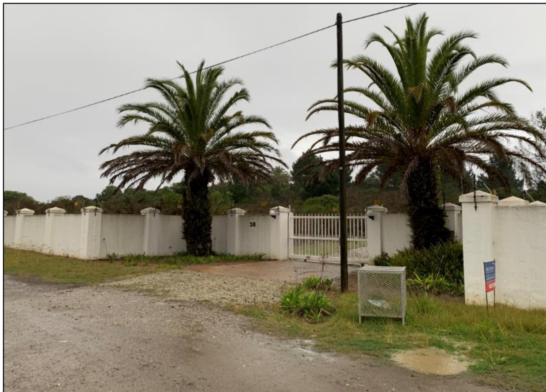
FIGURE 4: EXISTING ACCESS GATE
