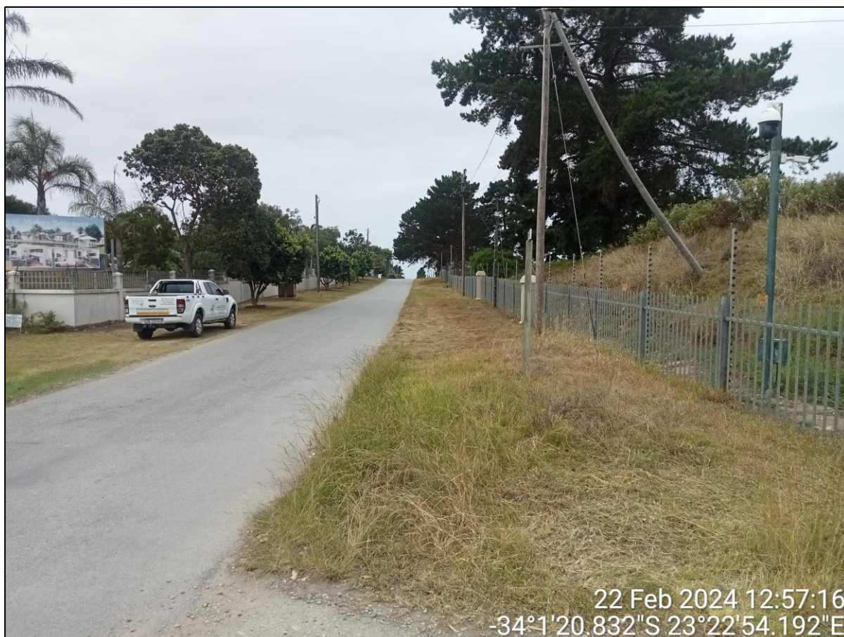
Figure 5: Rietvlei Road road reserve. Required sewage and water pipeline infrastructure to be installed within the road reserve.
