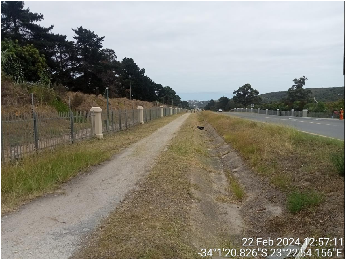
Figure 4: N2 road reserve. Required sewage and water pipeline infrastructure to be installed within the road reserve
