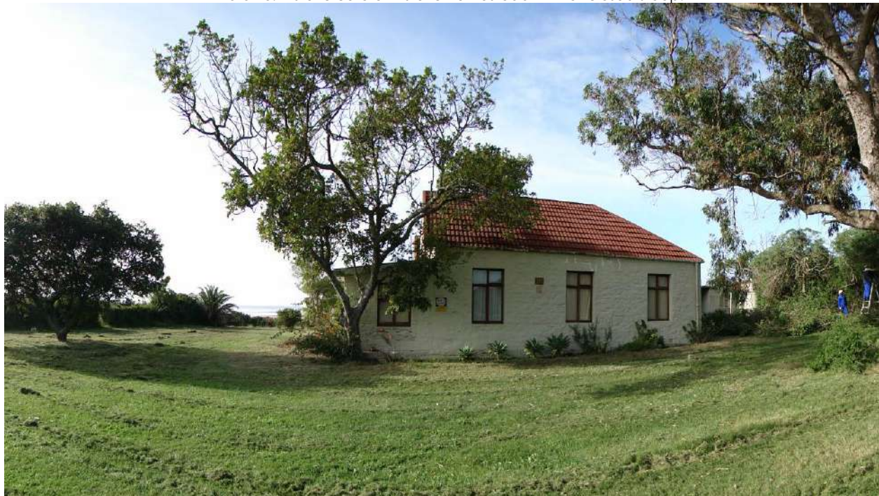
Photo 16: Northwest facing elevation of homestead. Stonewalling unfortunately painted.
