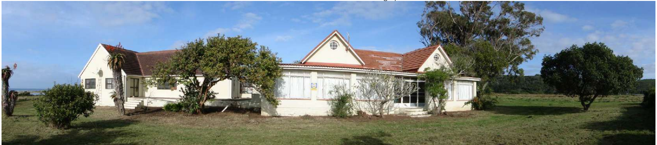
Photo 12: Northeast-facing elevation showing the historic homestead (right) and the modern home (left), which is physically connected to the historic homestead.
