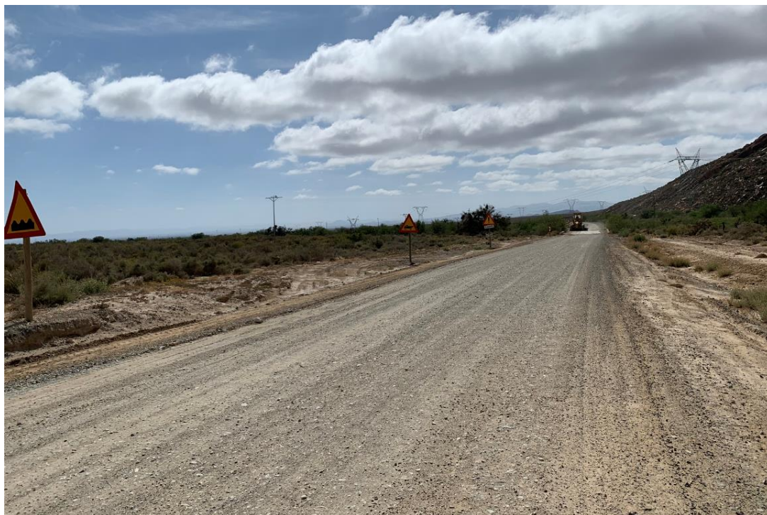
Figure A.9. Condition of the MR 319 / R356 to be used to access the site
