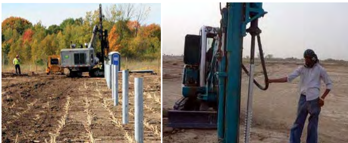
Figure 3: Driven/ Rammed Steel Pile (left) and Ground Screw (right) are the preferred mounting technology (Euphorbia PV, 2022)
