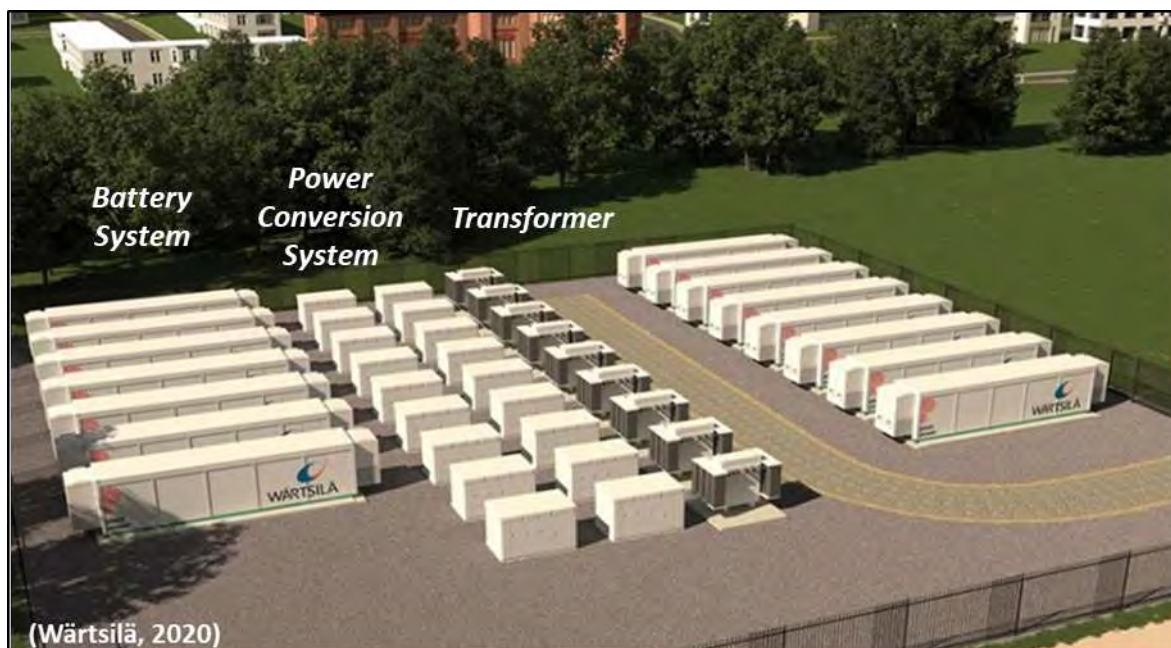
Figure 7: Pivot Power's proposed 50MW lithium-ion battery in Kemsley, Kent.
