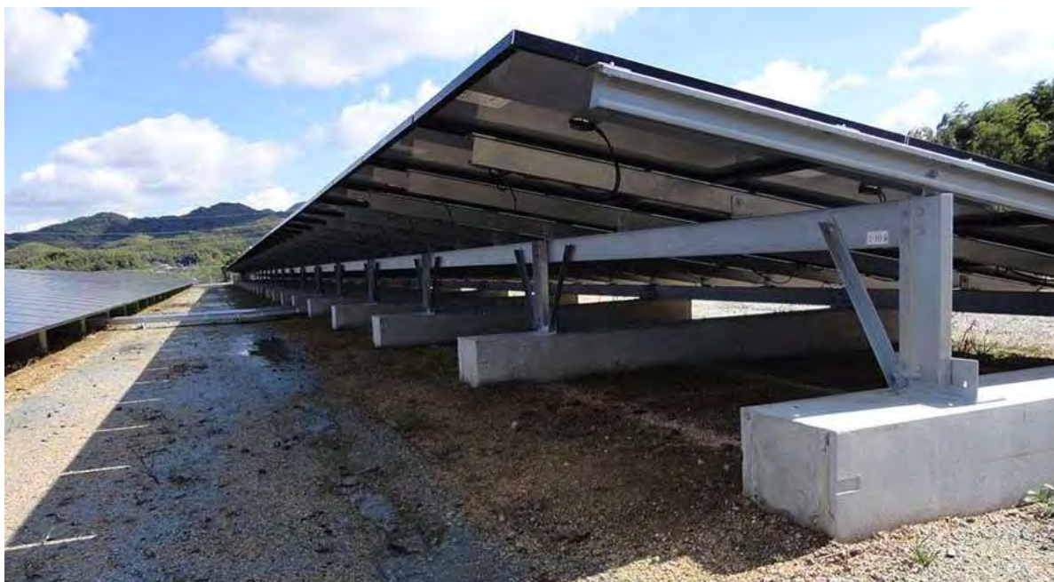
Figure 2: Cast Concrete Foundation - alternative mounting (Euphorbia PV, 2022)
