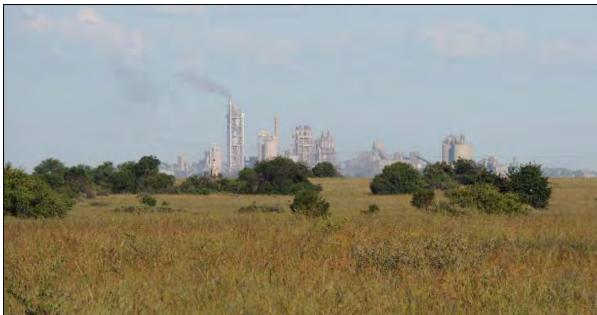
Figure 33. Photograph of the Lichtenburg LaFarge Cement Factory that forms a background view to much of the regional landscape (Stead, 2022)
