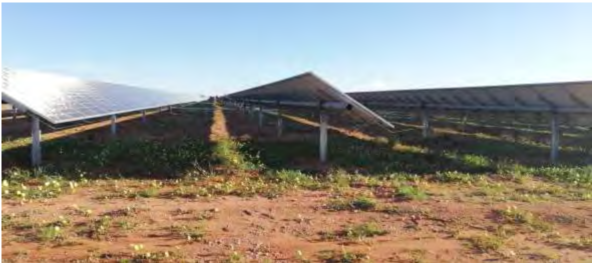
Single portrait module on a tracker (Photo – Cape EAPrac, 2019)
