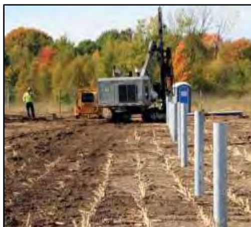
Figure 5: Driven/ Rammed Steel Pile
