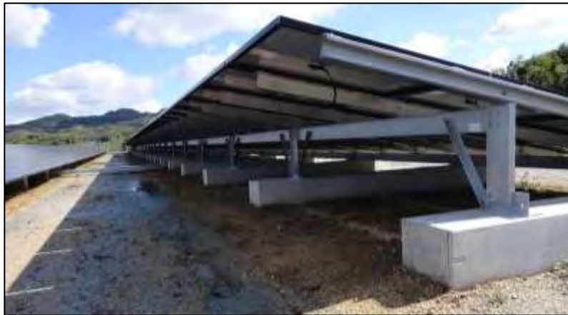
Figure 4: Cast Concrete Foundation
