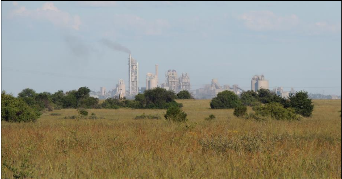
Figure 7. Photograph of the Lichtenburg LaFarge Cement Factory that forms a clearly visible feature in the regional landscape.
